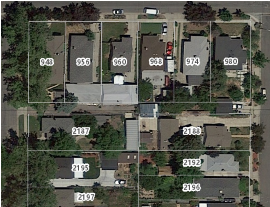
Figure 11 – In 2017, a different structure is visible on the west of the alley section.
